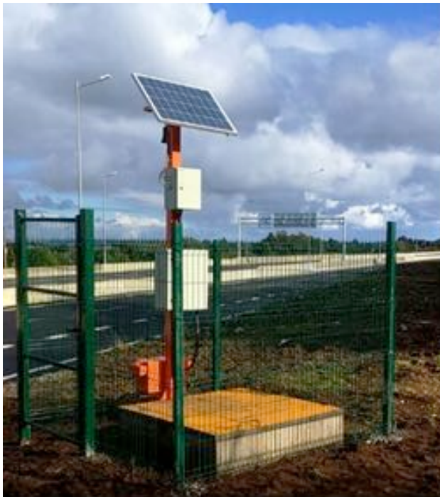
Typical solar power installation
