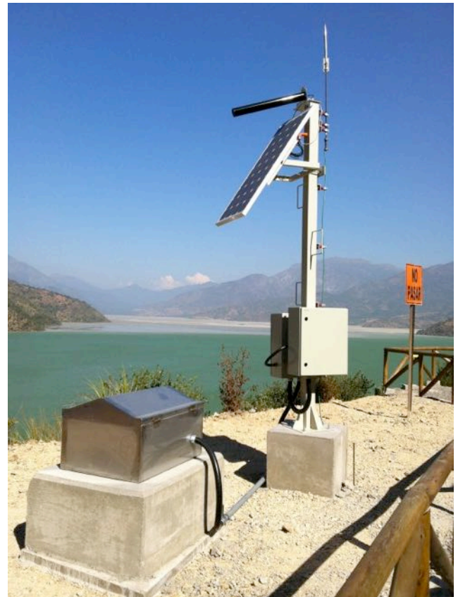
Typical solar power installation including lightning protection system
